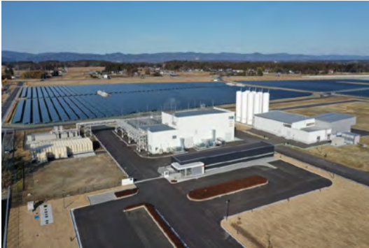
Picture 9: The FH2R facility in Fukushima. Photo: Toshiba ESS.
